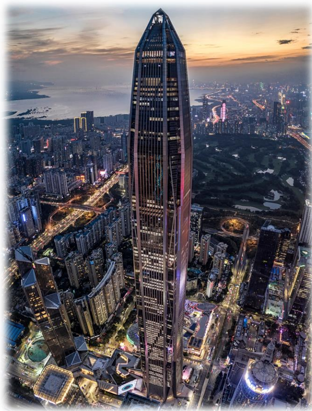
Ping an Finance Center in Shenzhen, China
